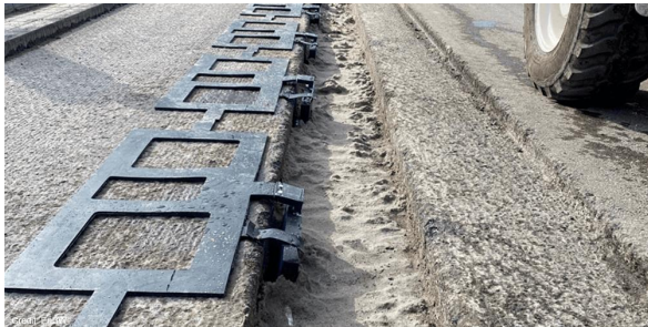
Fig. 1 Example of manually installed ERS transmitters
