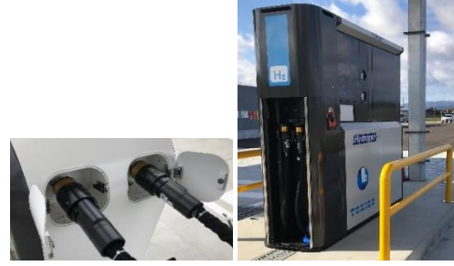
Fig. 4 Hydrogen refueling dispenser and nozzles at FTC
