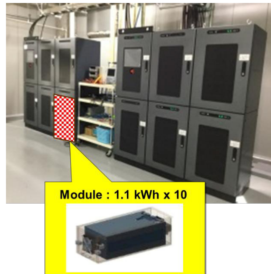
Fig.4 Photo of BESS installed SC-EIS function and assembled battery module
